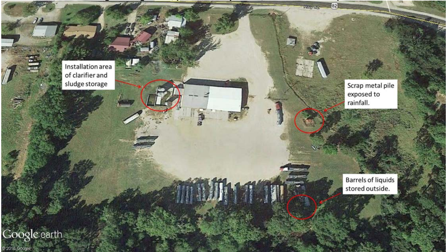
Figure 1. Overview of PJ'S Tank Wash in Crossett, AR. Locations identified are the installation area for the clarifier and sludge storage area, piles of scrap metal, and barrels of liquid stored outside.
